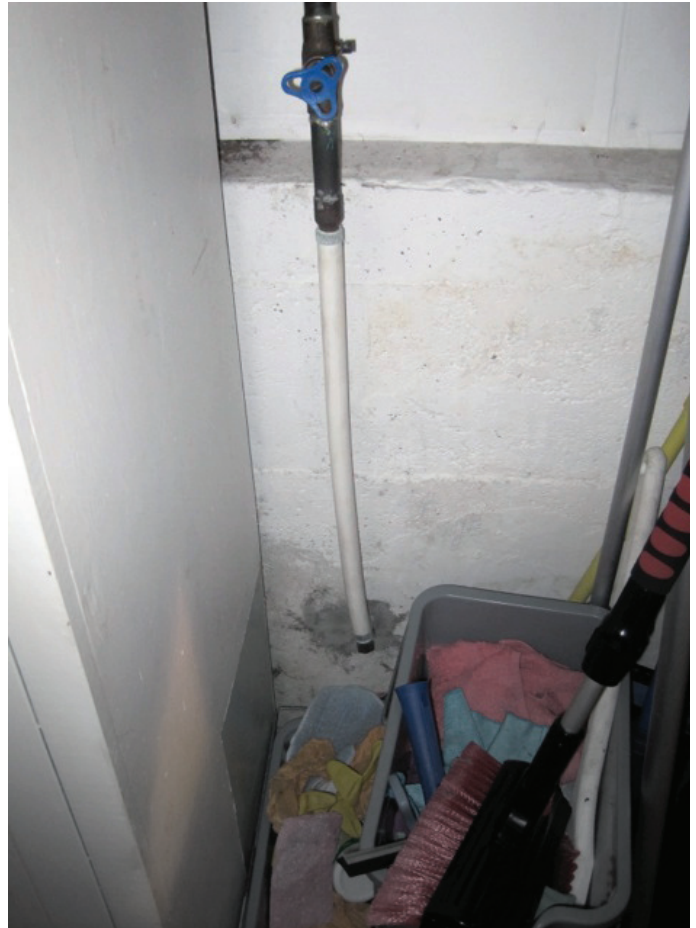
Broken ground due to water pipe repair with PEX
