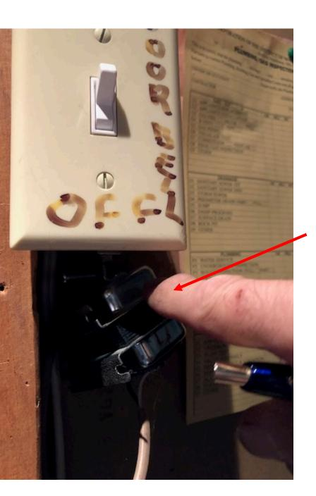
Doorbell installation incorrectly installed (doorbell transformer is ungrounded) – Common in houses pre 1960s:
