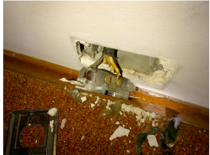
Ungrounded 2-prong receptacle fed by “modern” cable, NMD1
