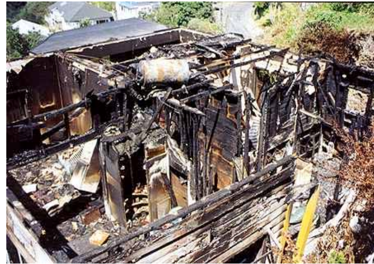
Aluminum-copper connections deteriorate over time, leading to fire
