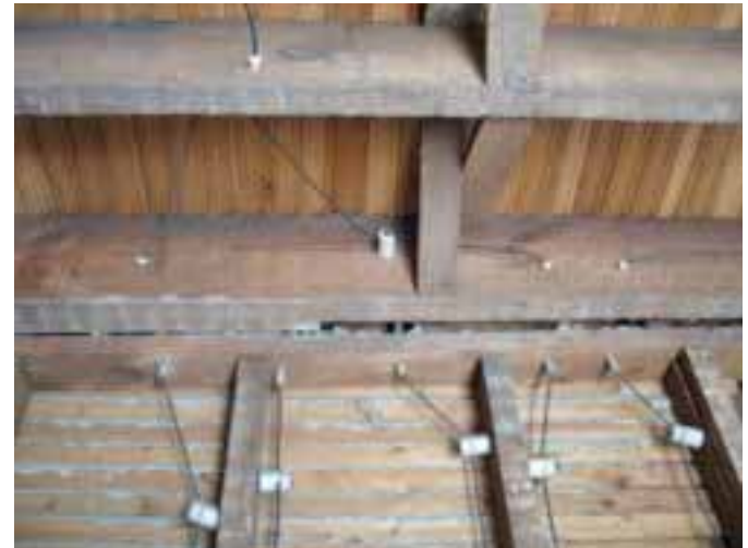
Typical Knob and tube wiring in a 1930s home
