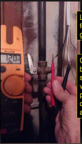
Live electrical conductor found millimeters from gas pipe
